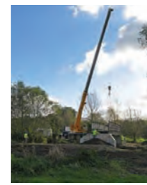
Construction of the new bridge. (Keith Hanna, Spokes.)
