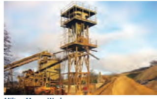
Milton Manor Works.
